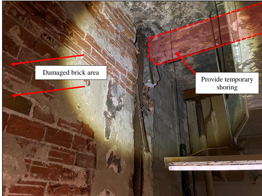
Photo 2 – Second Beam to Support
